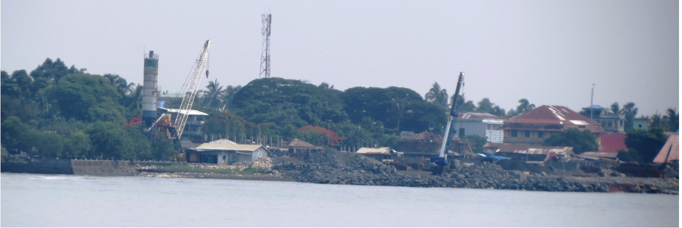
Under construction Sittwe Deep Sea Port 2014
